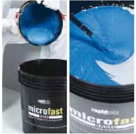
■ After 4-6 hours from the first coat, apply using a stainless steel spatula, the second coat of MICROFAST BASIC.
