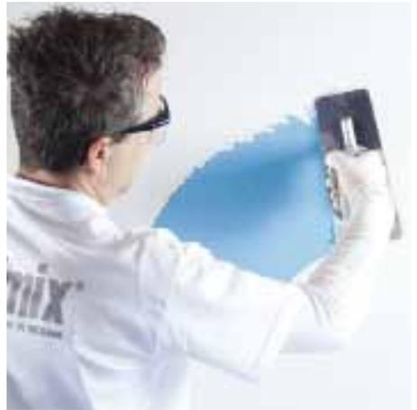
■ According to environmental conditions, wait about 4-6 hours before lightly sandpapering the surface using a 180-240 sandpaper.
