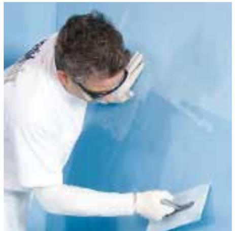
■ According to environmental conditions, wait about 4-6 hours before lightly sandpapering using a 180-240 sandpaper and remove dusts.
