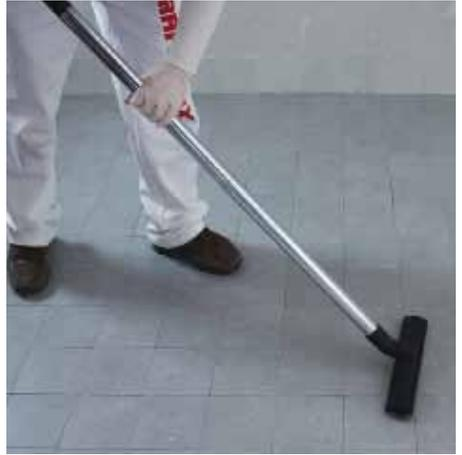
■ Put in the first layer of MICROFAST BASIC a 60-70 g/m<sup>2</sup> fibreglass mesh, and fix it with LATEX 200, applied using a long nap roller, with the 'fresh on fresh' method. Apply the first coat of MICROFAST BASIC with a stainless steel spatula.
